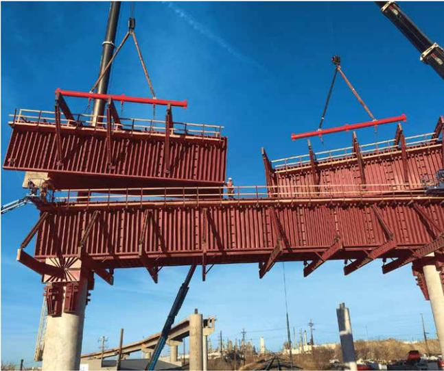
The Max-A-Form STS forming system is the Industry leader in rentable, self-spanning, steel formwork. Its superior pour pressure and moment capacities result in labor and material savings for the end user. The all-steel, welded frame make it the ideal choice for gang forming tall structural walls, pouring tieless columns, or for supporting concrete over long spans without shoring or custom equipment. The proprietary design and manufacturing process result in a superior finish, pour after pour.
