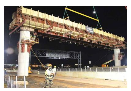
The Max-A-Form STS forming system is the Industry leader in rentable, self-spanning, steel formwork. Its superior pour pressure and moment capacities result in labor and material savings for the end user. The all-steel, welded frame make it the ideal choice for gang forming tall structural walls, pouring tieless columns, or for supporting concrete over long spans without shoring or custom equipment. The proprietary design and manufacturing process result in a superior finish, pour after pour.
